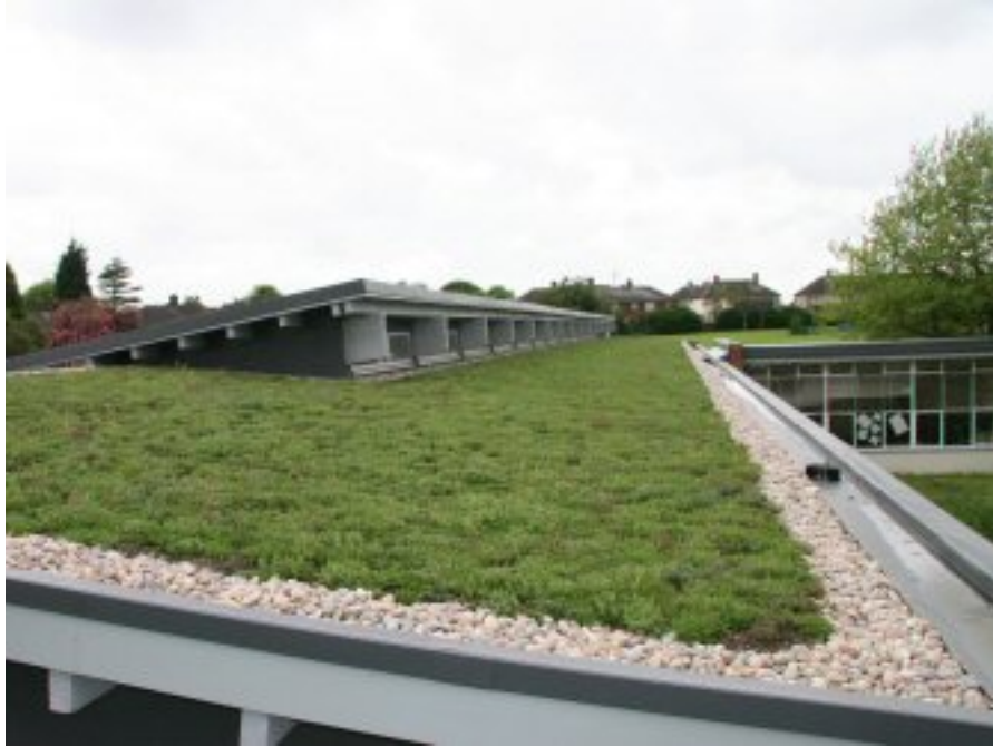
Figure 5a. Green Roof for Lower Building Maintenance Costs
