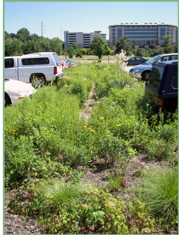
Figure 7. Vegetative Swales and Medians
