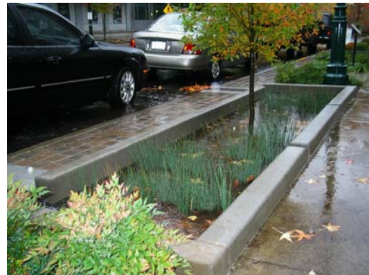
Figure 9. Infiltration Planters
